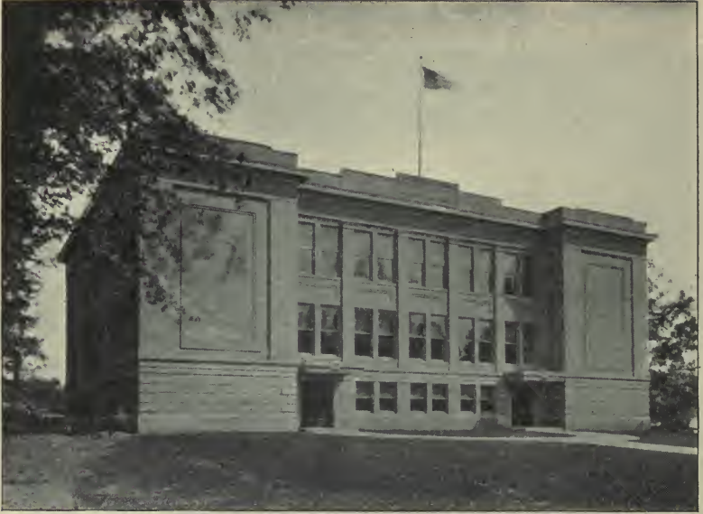
Public school building at Sherman, Chautauqua county
